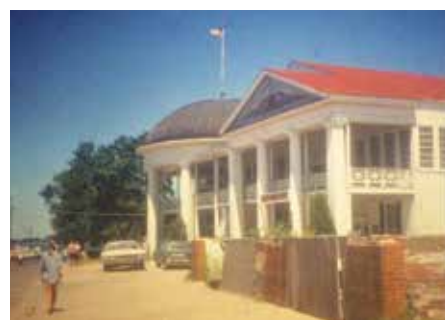
These remains of the front of Schnoor and Fuch store show just how close the building was to the old Colonial.
